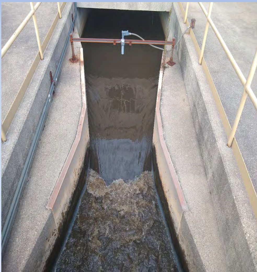
Headworks – Parshall flume measuring influent flow
