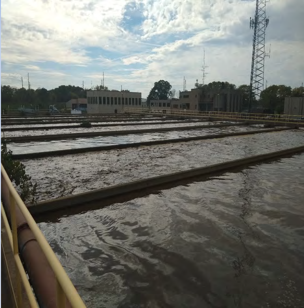
8.4 million gallon oxidation ditch with 4 aerators
