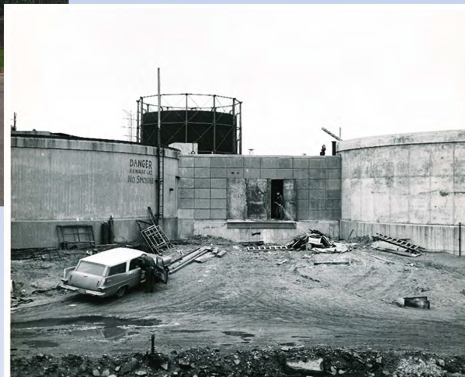
Dewatering building –3 sludge holding tanks, originally constructed in 1940's
