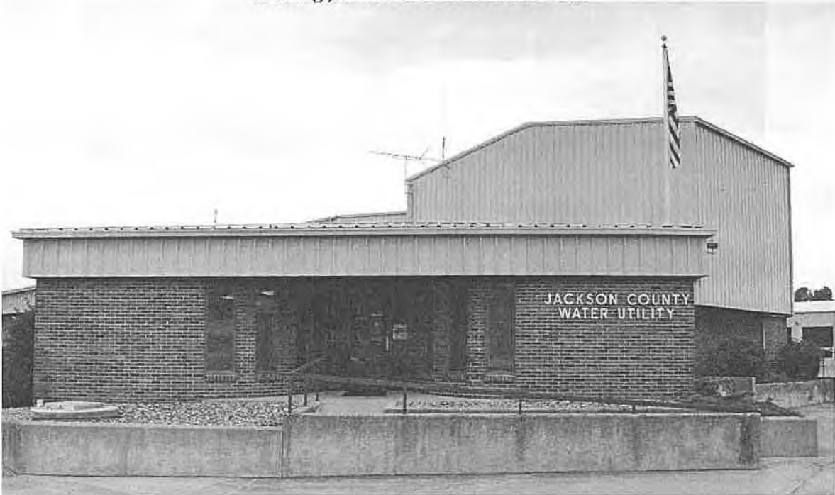
Existing JCWU Water Treatment Plant
