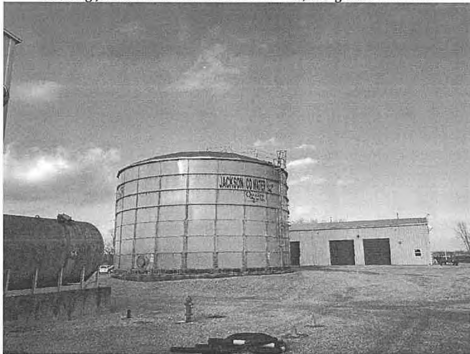
Existing JCWU Water Treatment Plant 750,000-gallon Clearwell
